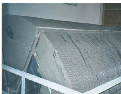
Figure 6. Construction of the RBC units.
